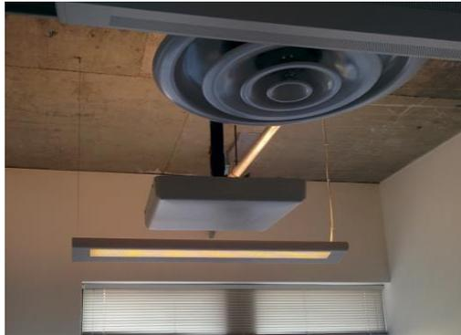
*The xArray is slightly below the vent and lighting to avoid interference*
